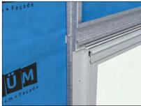
Install the horizontal trims for the cladding, at the top and bottom of the cladding section, above and below any wall penetrations, and at any slab junctions.
